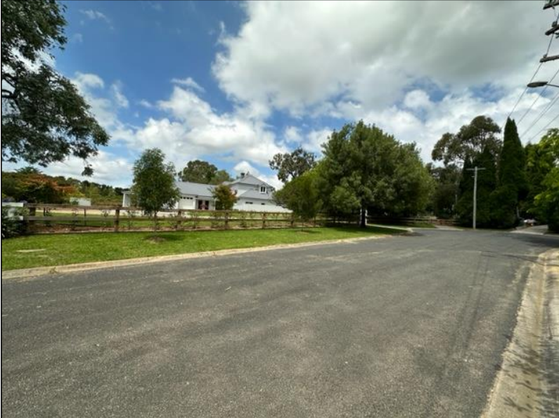
Figure 10: View of 35 Elizabeth Street
