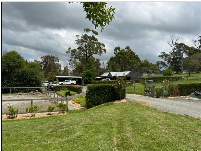
Figure 7: Existing farm buildings on 4 Old Bong Bong Way
